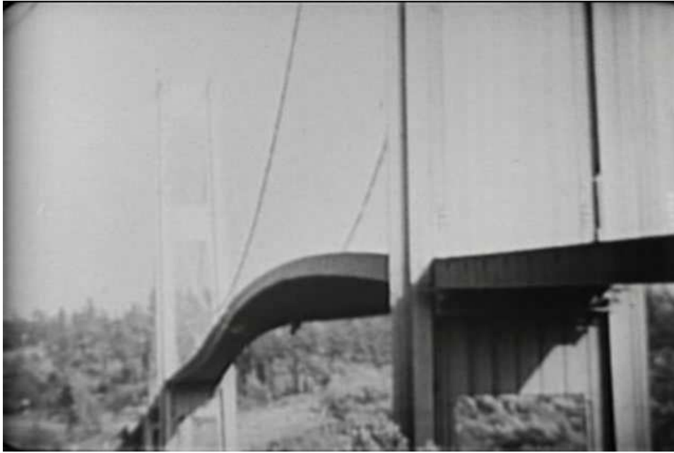
Figure 1.5: Tacoma Narrows moments before the collapse.
