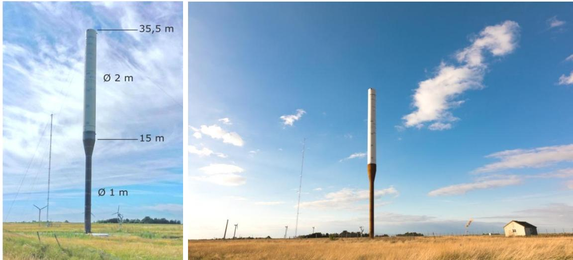
Figure 1 Views of the chimney and the wind mast
